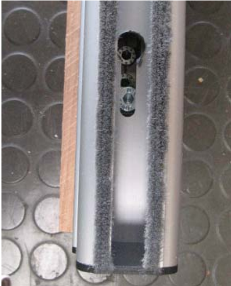
Fig. 7 Fixing of height compensation profile with top rail
