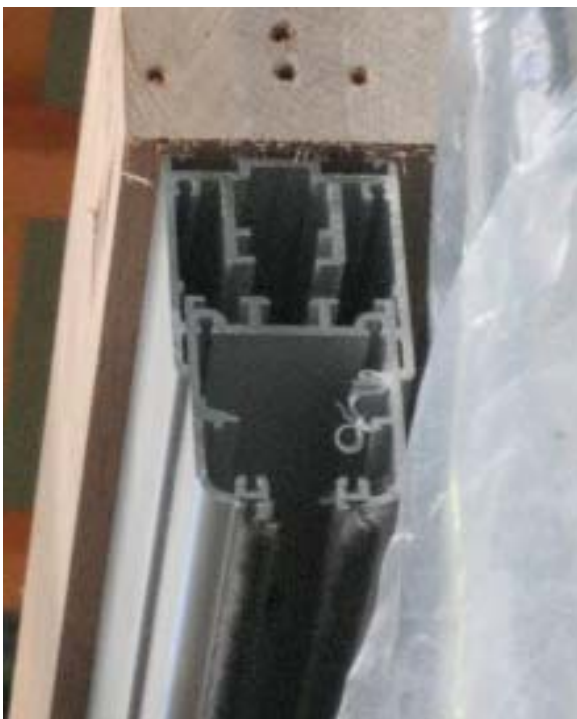
Fig. 5 Top rail in height compensation-profile (without end cap)
