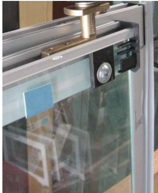
Fig. 10 Support of pane (cover section removed)
