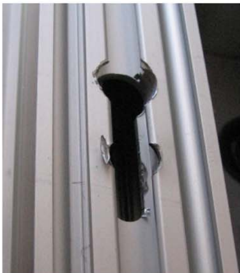
Fig. 2 Cause of failure, break-outs at Aluminium profile around screws.
