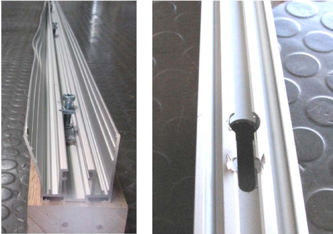
Fig. 2 and 3 Cause of failure, aluminium profile torn out around screw heads
